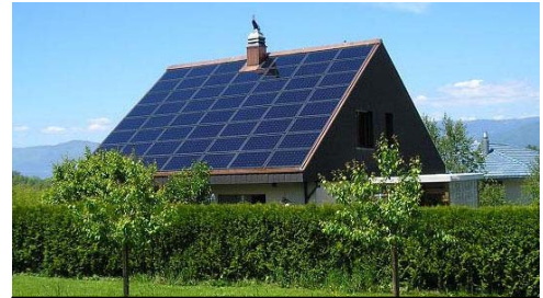
Example of a Solar Conversion System, Structure-mounted
