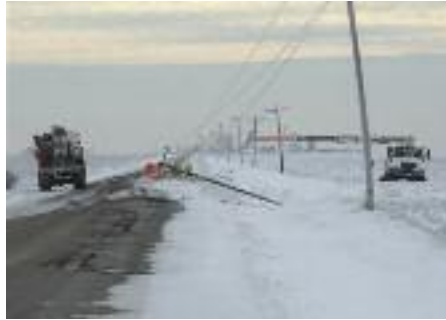
Strong winter winds can cause ice to build up on one side of a power line, causing them to bounce.
